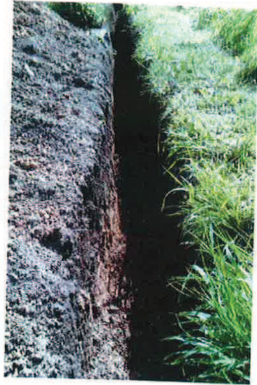
New trench for the water pipe.
